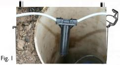
Splice wires using supplied crimp connectors.
