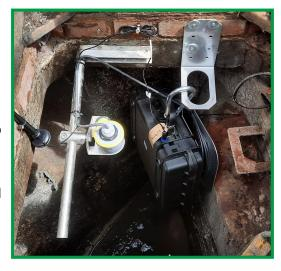
Intelligens WW was the obvious choice for this level monitoring application. It is used in-conjunction with an external battery which also powers the connected sensors, making it particularly suitable for 'fit and forget' long-term installations.
