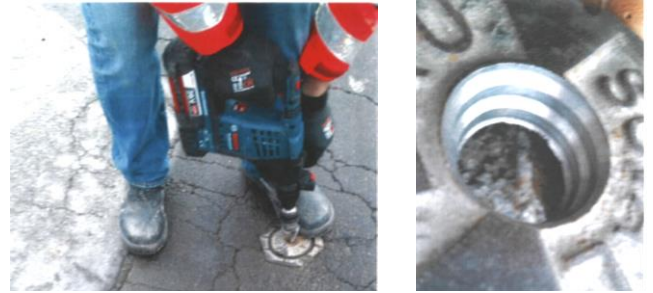
Figure 19. Drill hole and recess in chamber lid
