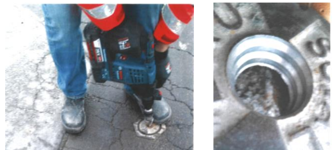
Figure 20. Drill hole and recess in chamber lid
