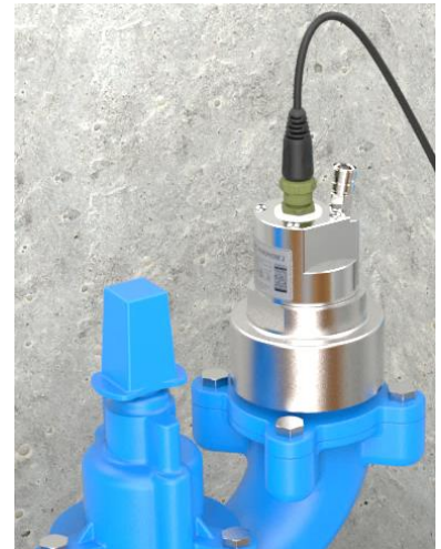
Figure 18. Example of a Hydrophone-2 installation
