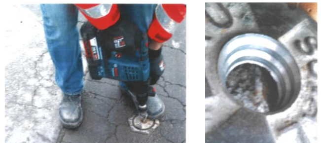
Figure 20. Drill hole and recess in chamber lid
