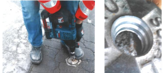
Figure 31. Drill hole and recess in chamber lid
