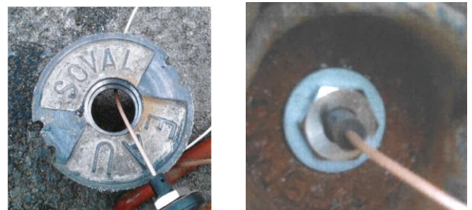
Figure 32. Thread antenna into position and secure in place with supplied nut and a suitable washer
