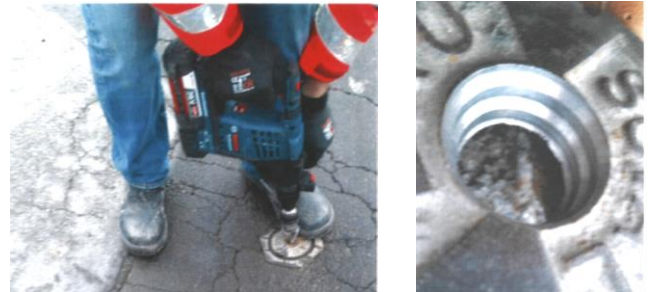
Figure 32. Drill hole and recess in chamber lid
