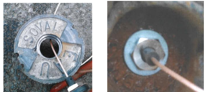
Figure 33. Thread antenna into position and secure in place with supplied nut and a suitable washer
