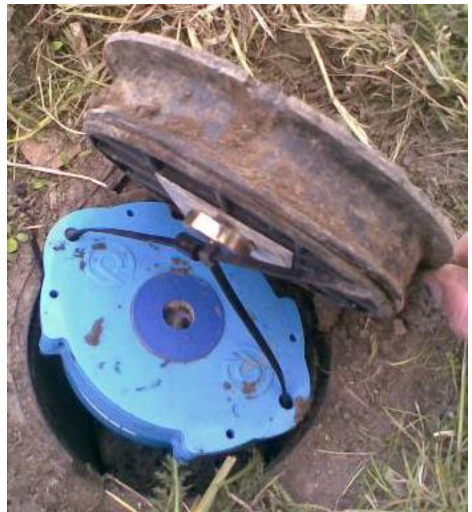
Figure 17. Logger in Talbot flip-lid box P-clip example
