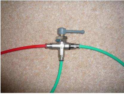
To override the Pegasus+ controller and place the PRV into a fixed outlet pressure, at the maximum pressure set on the actuator turn the handle on the 3 way tee 180 degrees to point the handle at the red pipe. This will give a 24/7 fixed outlet pressure.
