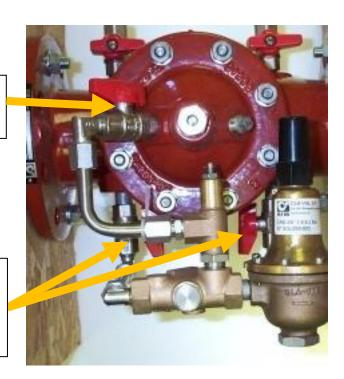
Note: The upper chamber of the PRV valve is now locked in position.
