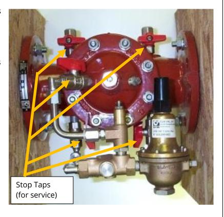
Lock the PRV top chamber by closing the valve to the top chamber, if possible.
